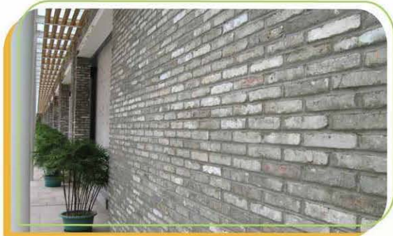
售票處外的磚牆是利用回收的青磚砌成 Reused Chinese bricks are used for building brick wall outside the ticket office
