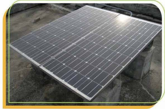
濕地保護區內觀鳥屋裝置了太陽能光電板 Photovoltaic panels are installed in bird hides for oscillating fans
