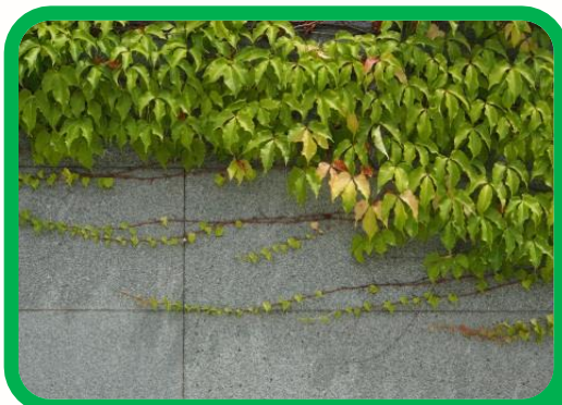
Wall covered by climbing plant
